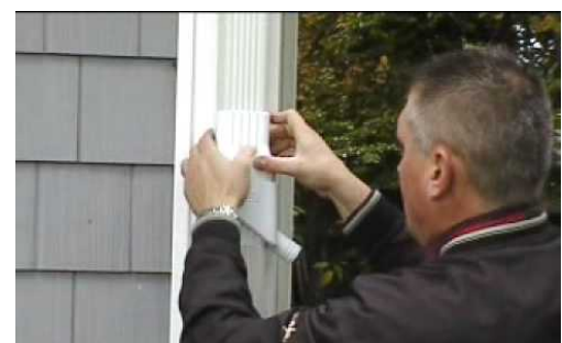
Resident Installing Diverter
